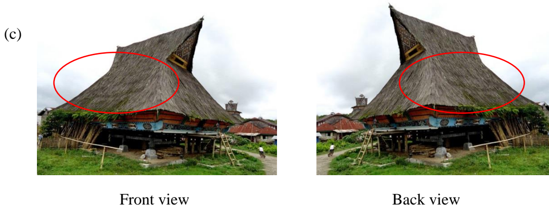
Figure 8. Roof of Karo Traditional House
